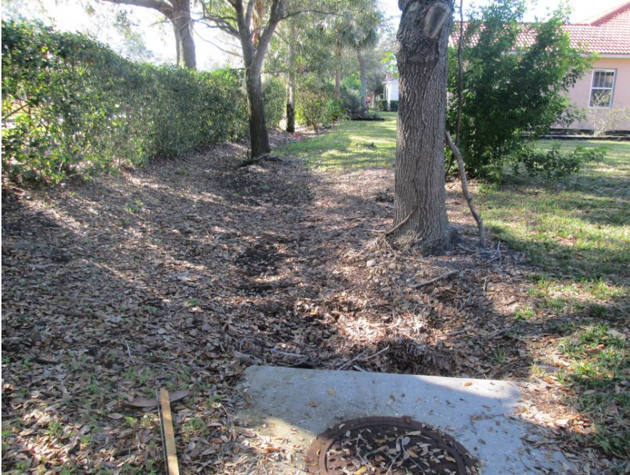
Viewing swale from inlet at Dry Retention Pond viewing south
