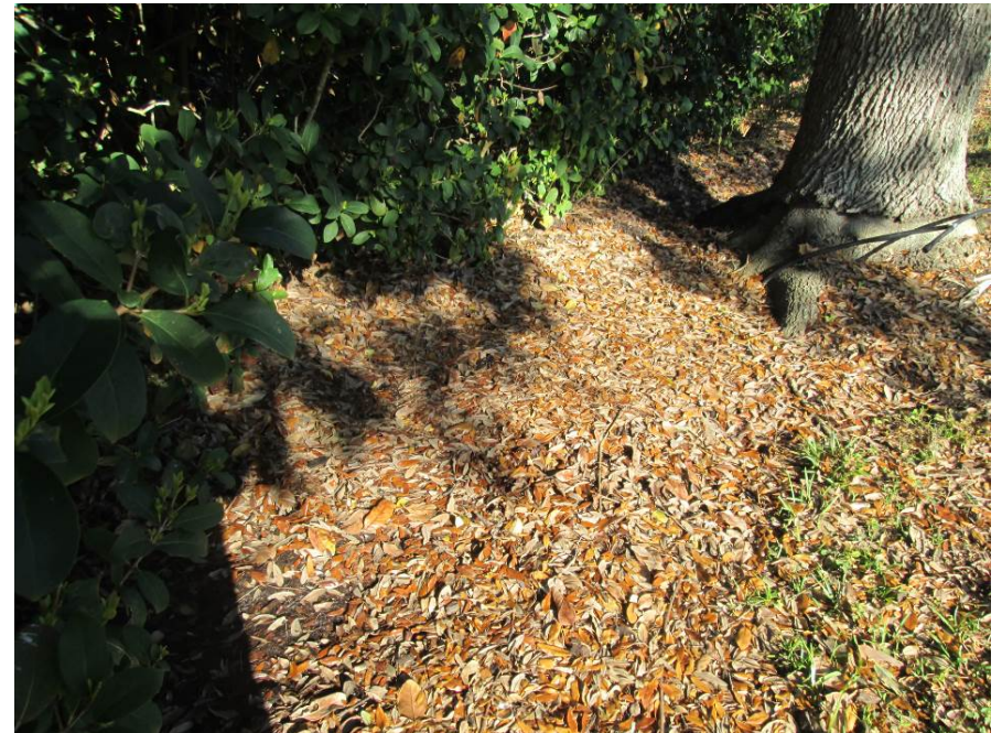
Tree growing along edge of swale impeding flow from swale
