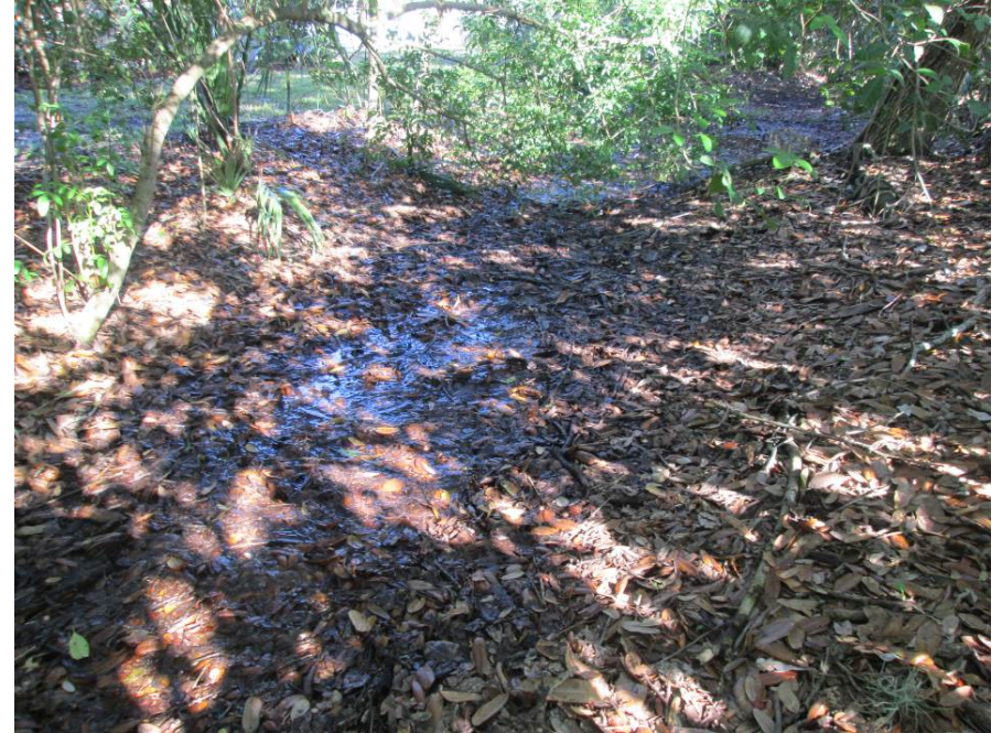
Standing water in swale behind middle section of Skyward Ct
